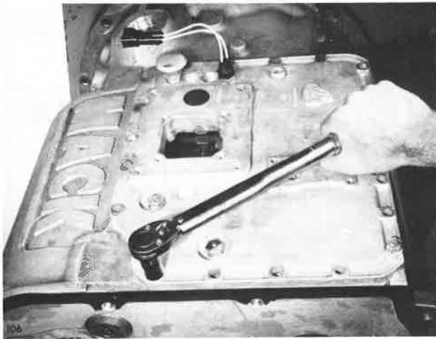
Tightening Top Cover Capscrews
